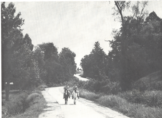
A VIEW OF THE FIRST CONCRETE ROAD SOUTH OF OHIO RIVER—U. S. 45 IN LEE COUNTY, MISSISSIPPI
